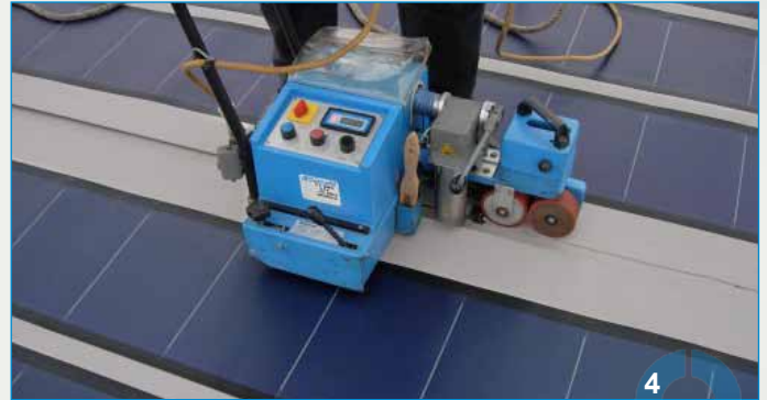
Welding with automatic equipment
