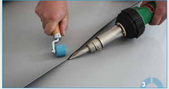
Welding with manual equipment
